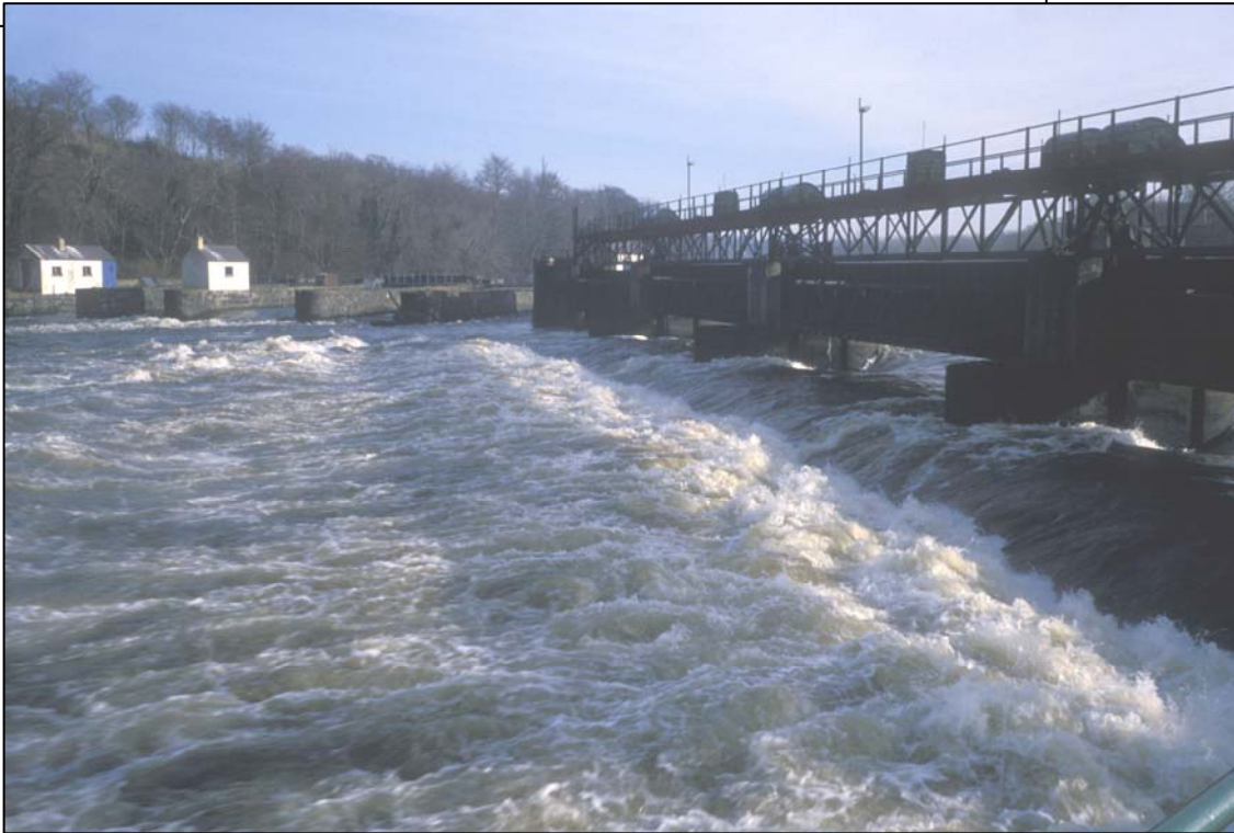
Plate 4 - Sluice gates and their position along the Bann corridor
